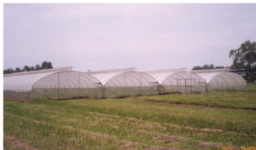
Plate 2: Quadruple-span greenhouse structure
