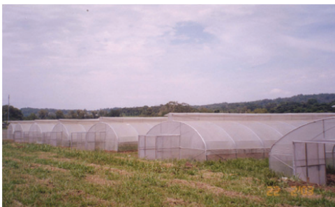
Plate 1: Single-span greenhouse structure
